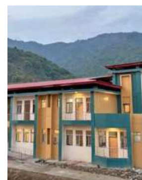
The foundation of the institute, located in Jote, was laid by the Prime Minister eight years ago.
