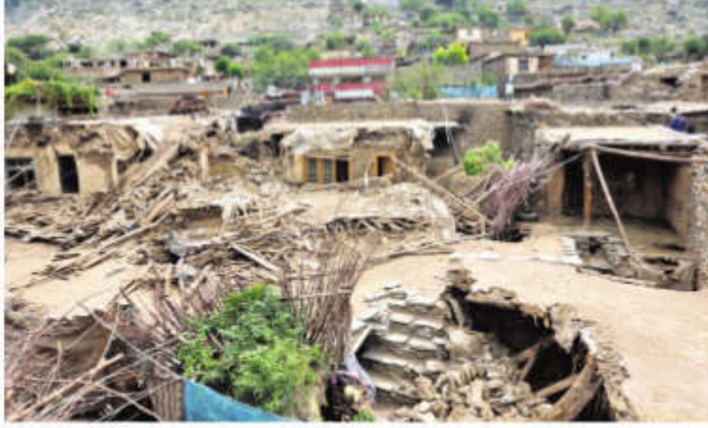
Collapsed houses in an area devastated by powerful earthquake that killed many and destroyed villages in eastern Afghanistan in Kunar province | AP
